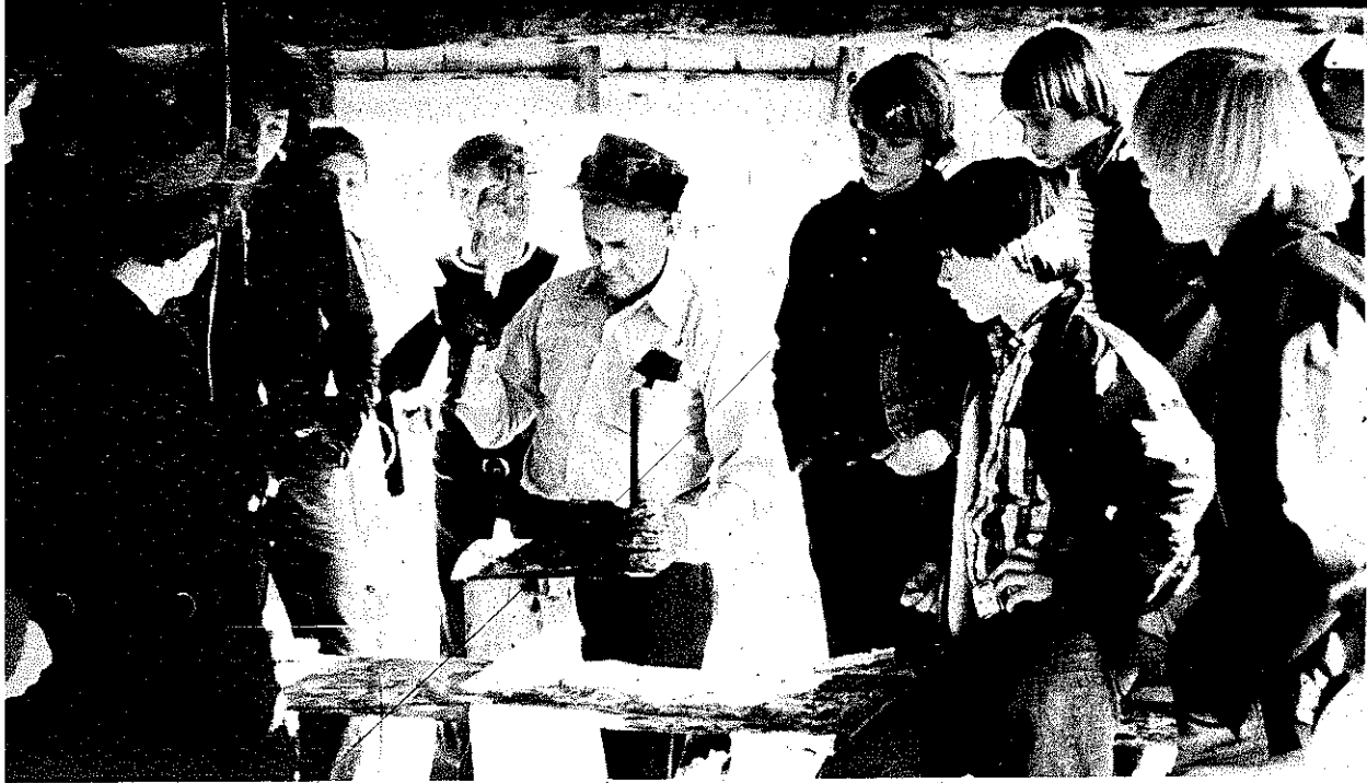
PLATE 311 Foxfire editors watch as Woodrow splits the white oak boards for covering the roof.
