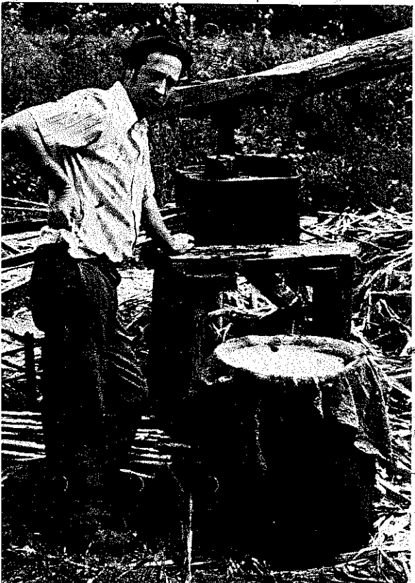
PLATE 419 The burlap bag spread over the barrel serves as a strainer. This is the first of three strainings during the entire sorghum-making process.
