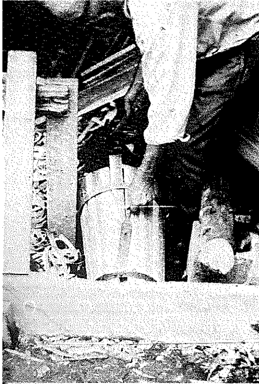
PLATE 348 A chisel can be used as shown to help fit the last stave.
