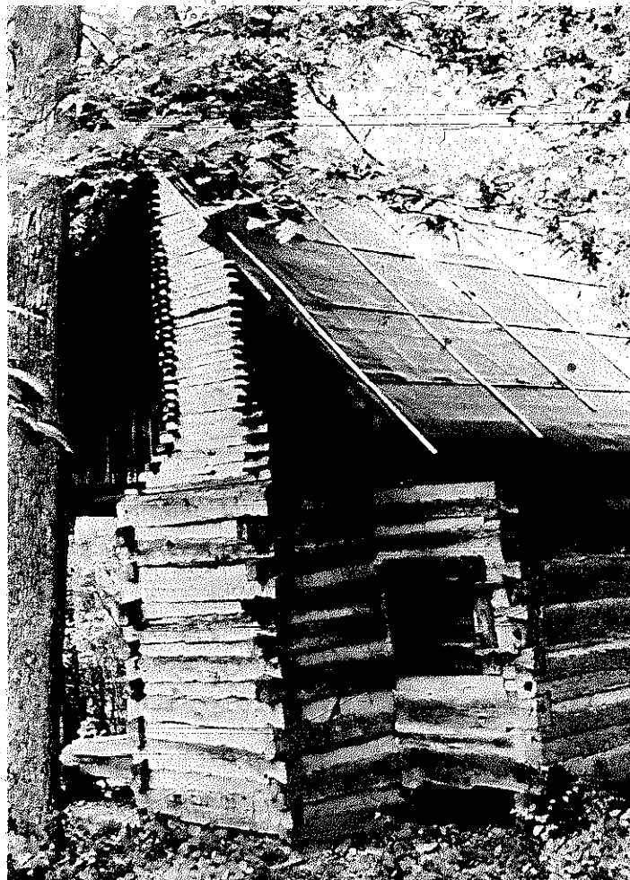
PLATE 372. A beautiful stick-and-mud chimney on a cabin near Brasstown, North Carolina. Note also the gable of hand-split shingles and the wooden shutter with wooden hinges covering the window. Such shutters were used in place of glass, which was not available at the time.
