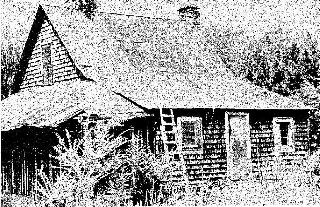
PLATE 141 A house near Tallulah Falls, Georgia, covered with shingles.
