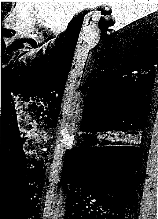
PLATE 189 The backs fit snugly into the slots just cut for them. Lon shapes the top corners (arrows) for decoration.
