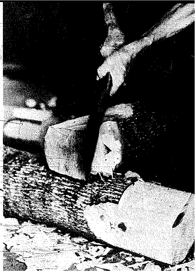
PLATE 71 Turn the log over as necessary to accomplish hewing.
