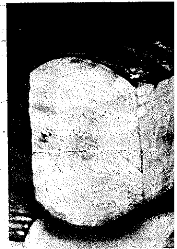
PLATE 63 The two sides hewed, the log is now ready for notching. The remainder of the sides will be hewed after the logs are all in place in the cabin.
