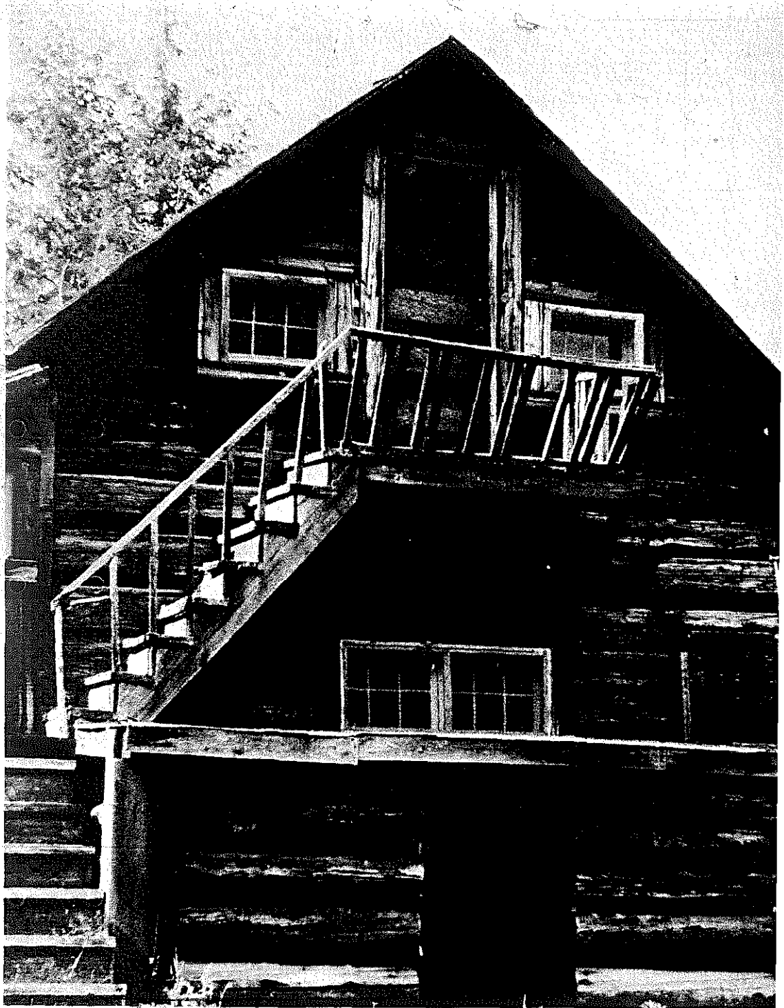
PLATE 123 The gable can be designed to hold a door and windows, as seen on this cabin at the Jay Hambidge Art Foundation in Rabun County.
