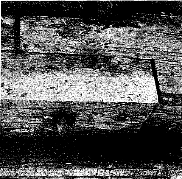
PLATE 92 Two logs were hewn and lap-jointed together to make this plate. A wooden peg through the joint ensures that they will not slide apart.
