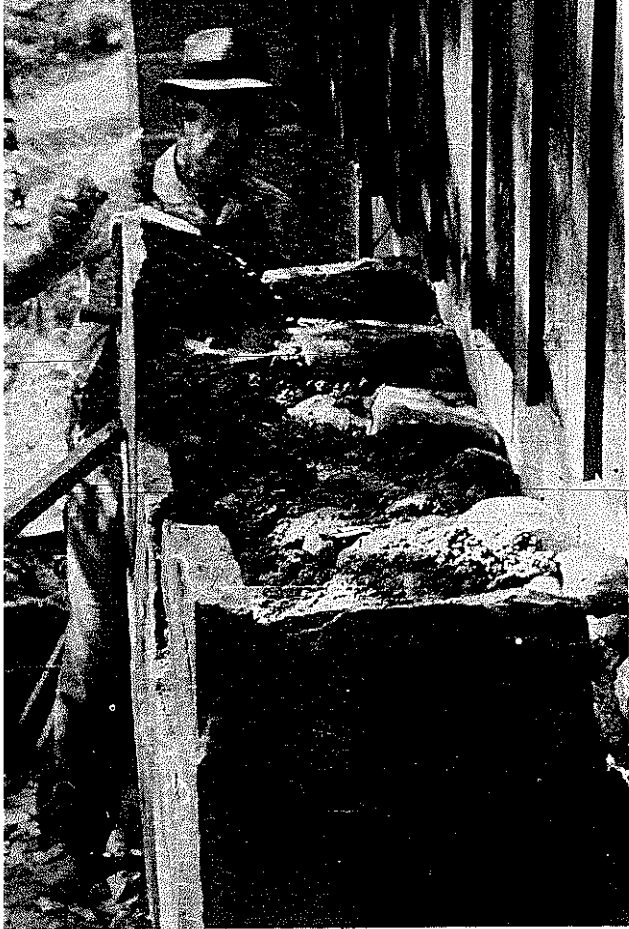
PLATE 148 Claude Darnell, a master chimney builder, often faces his chimneys with flagstone. The flagstone is cemented in place a round at a time, and the box thus created is filled with a "stuffing" of creek rocks and cement.
