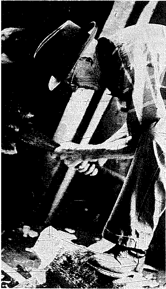
PLATE 81 Harley Thomas demonstrates another method for cutting the same notch. Hew a peak as above.
