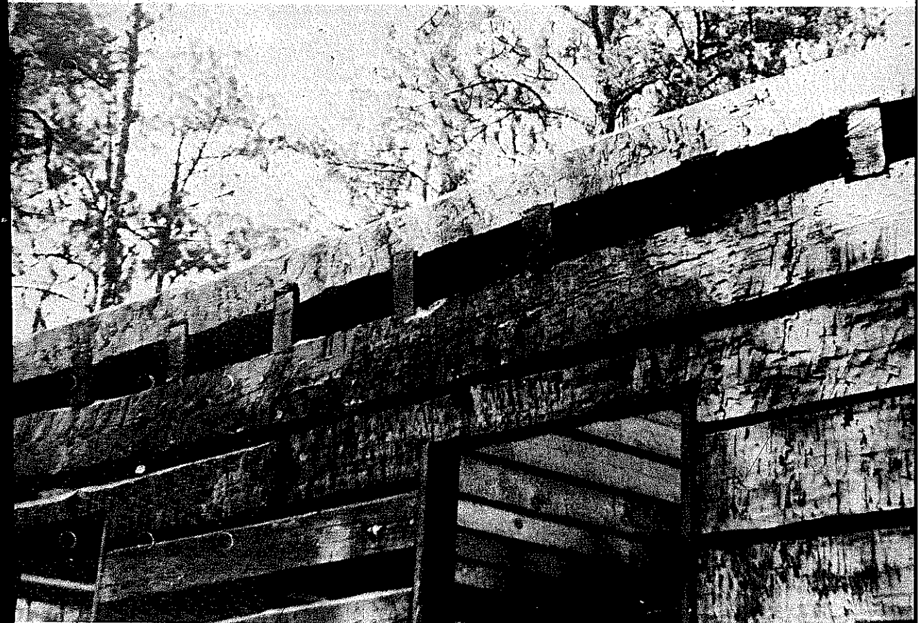
PLATE 100 In the South Carolina reconstruction, both the plate and the log above it are notched to fit the joists.
