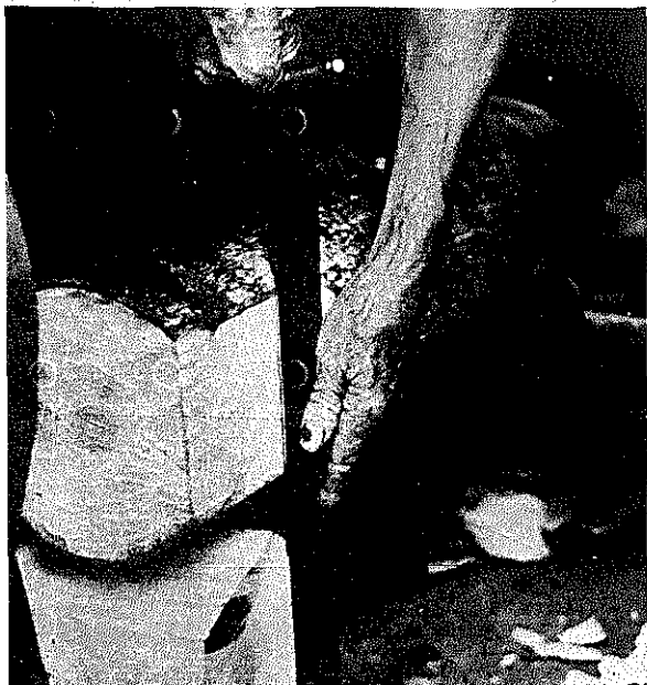
PLATE 68 Now, placing the ruler as shown, draw a vertical line on the top log which intersects with the sloping line.
