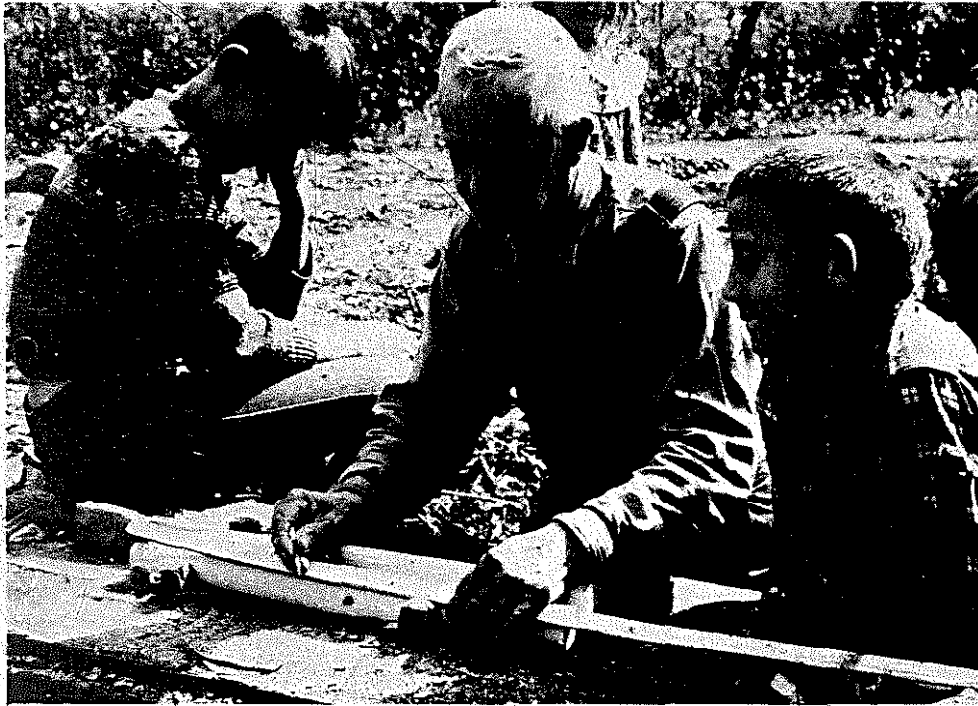
PLATE 190 The short legs are now marked for the placement of rounds.
